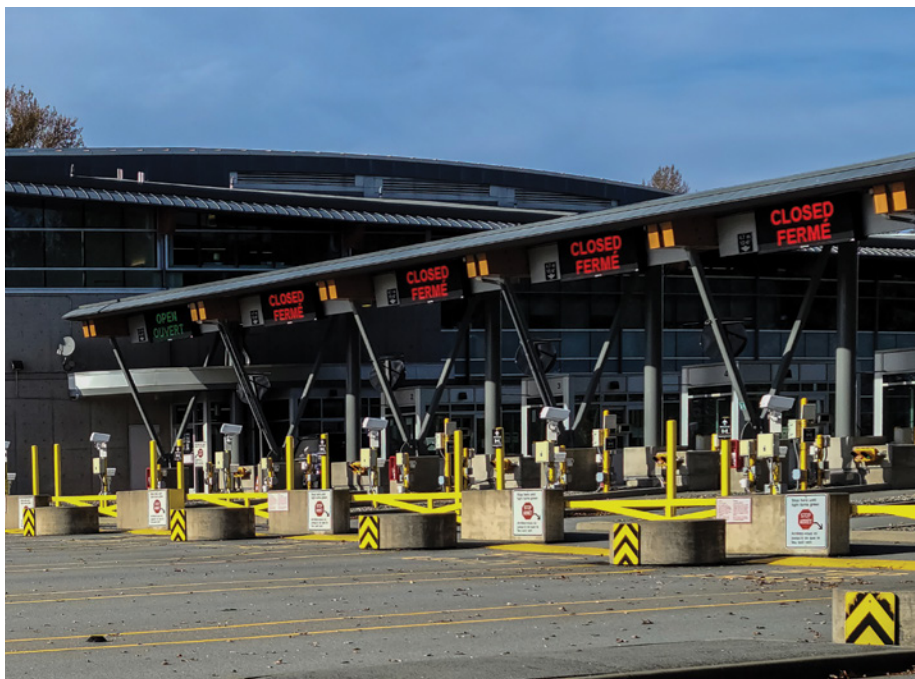
The B.C.-Washington State border crossing south of Vancouver, in normal times, one of the busiest land crossings between Canada and the US, but bereft of non-essential traffic for the 18 months of closure due to the pandemic. iStock photo
