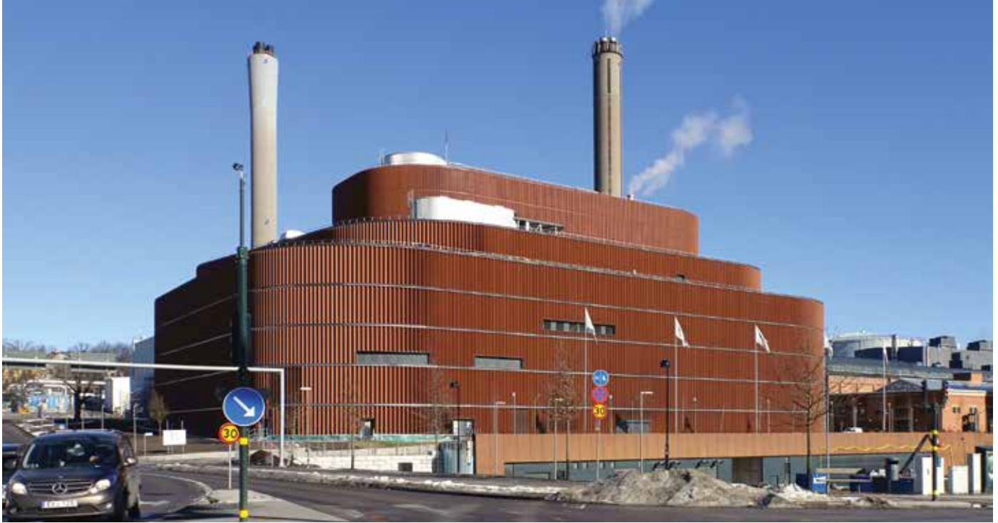
The wood chip-fuelled KVV8 combined heat and power plant in Stockholm heats 190,000 residences and generates enough electricity for 150,000 electric vehicles, with lower air pollution emissions intensity than a natural gas furnace. — Holger.Ellgaard
